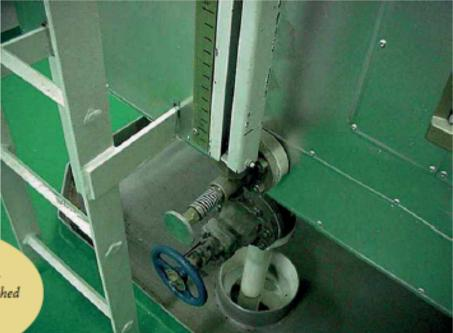
In the event of a fire, the plastic tubing will melt. With the self-closing valve lashed back, the tank is open to feed the fire.
